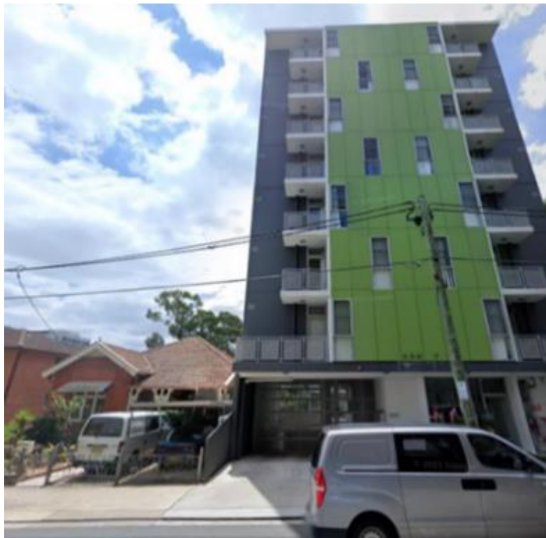
Examples of interface sites and the built form outcomes that will be enabled by the proposal
