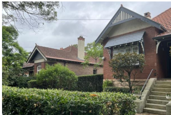
Typical historic built form and gardens in the affected heritage conservation areas.
