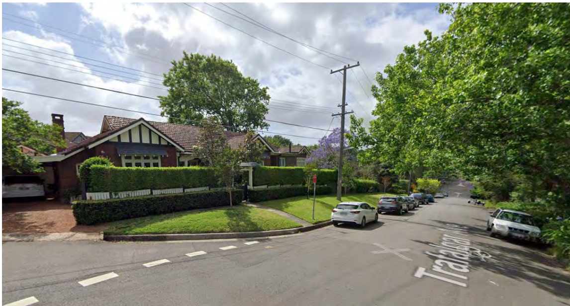
Above: Trafalgar Avenue, Roseville conservation area proposed for 6-7 storey apartments
